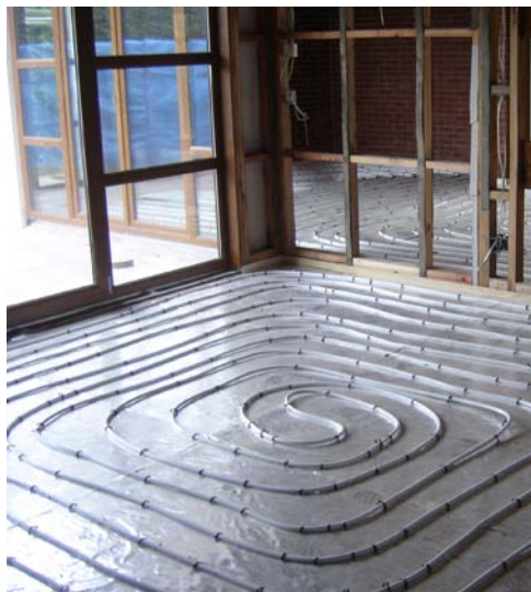
A NZ screed underfloor heating system during installation.
