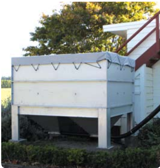
Wood pellet storage hopper.
