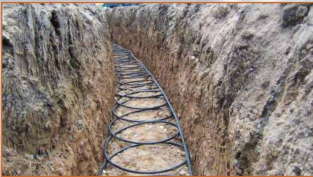
The 'slinky' pipes laid in the trench.
