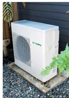
Air-to-water heat pumps are electric appliances that heat the water that circulates through a central heating system. The air-to-water heat pump converts large amounts of low temperature heat in the air to small amounts of high temperature heat.
