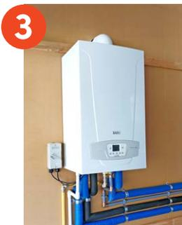
Boilers burn a fuel to create the high temperature water for circulation through the heating system. Diesel boilers are more common in the South Island while gas boilers are popular in the North Island where reticulated gas is available.
