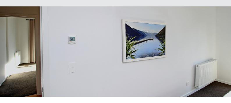
in sun hours between different parts of the home will result in very different heating needs. When reviewing the plans for a home, our engineering team will consider these factors, and where required, additional control zones will be added to the system to help manage these varied heating needs.
