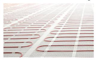
An electric underfloor heating system consists of electric heating cables being installed beneath the floor. Electricity is then passed along the resistive cables causing them to heat up and radiate the heat into the room.
