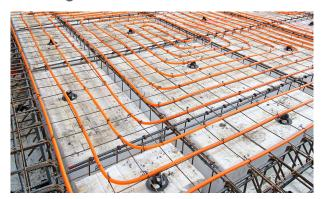
Hydronic central heating is a method of whole-home heating in which warm water circulates through a closed network of pipes, carrying heat around the home. The heat source warms the water circulated through the pipes that lead to the pipes laid in the floor for underfloor heating. Ideal for whole-home heating.
