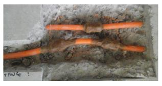
Following the repair of the damaged pipes the system should be put back under pressure test and hold pressure for 24 hours before the exposed pipes can be backfilled. Location of the repairs should be recorded and shown on as-built drawings for future reference. From our experience these repairs will have a long life but are the most likely location for any issues in the future so being easy to locate would be preferable.
