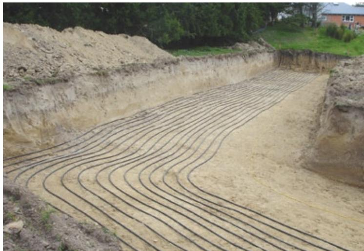
bottom of a wider trench. The trench lengths are likely to be 20-30 percent of the length of a single pipe configuration, but the pipe length may double for the same thermal performance.
