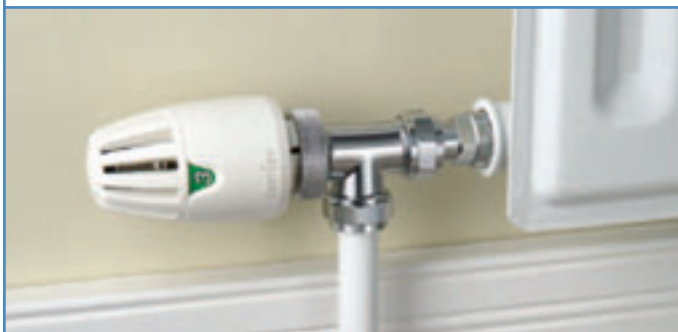
Terrier TRV fitted horizontally at bottom of radiator
