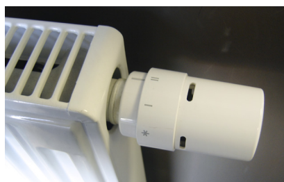
The radiator valve (TRV) allows for individual temperature control on each radiator
