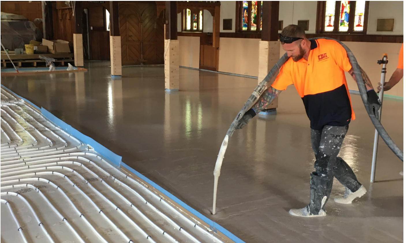
EzyMix being poured over underfloor heating piping at Nelson's All Saints Church
