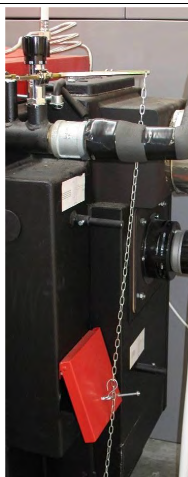
Air flap in approximate boiler off position. Chain below flap not attached to anything.
